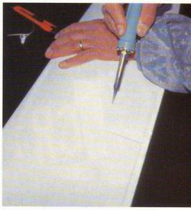
Alternatively, if the control surfaces are 'living' hinged with nylon ribbon during the construction (as is often the case today), cut the vinyl at the hinge gaps and at each extremity. Then apply the tip of your soldering iron along the control surface slit whilst taking care to operate the control surface in order to widen the slit. Repeat the operation two or three times.
